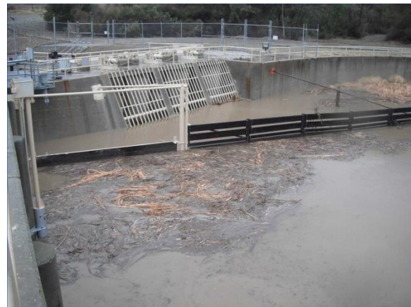
Figure 6. Timber Debris Fence and Trashrack Looking Downstream
