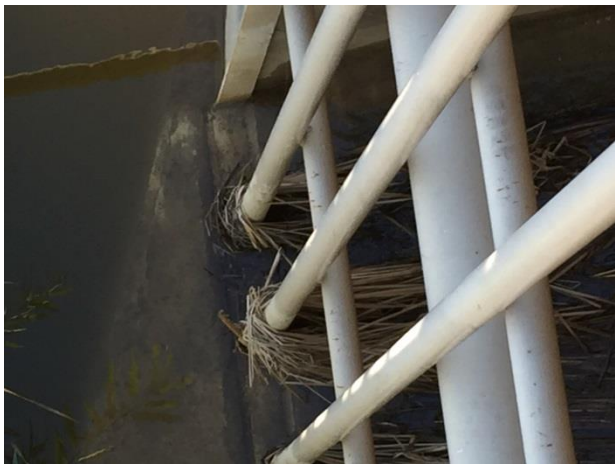
Figure 14. Grasses on Coarse Trashrack
