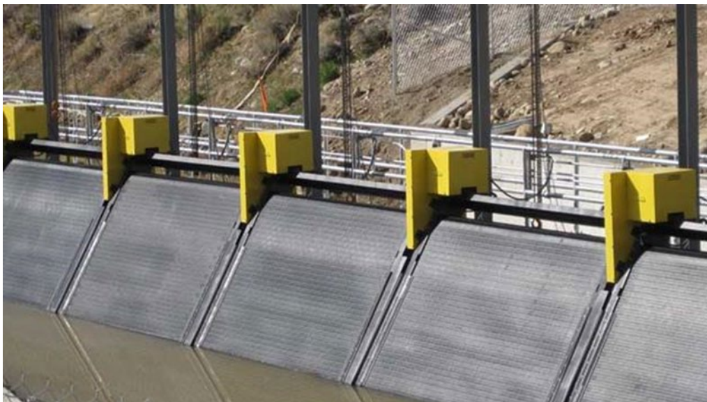
Figure 3-8: Angled Hydrolox Screens at the Ray Canal Diversion on the Little Wind River, Wyoming (Courtesy Hydrolox)
