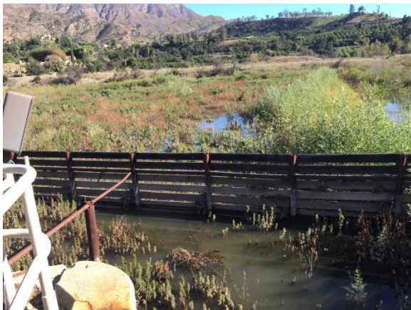
Figure 5. Timber Debris Fence Looking Upstream
