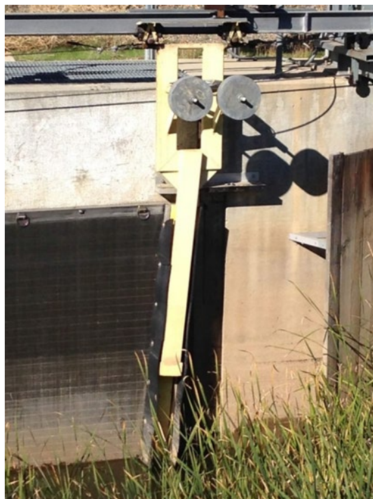
Figure 3-3: Existing Robles System, Single Brush Arm with Two Closely-Spaced Brushes
