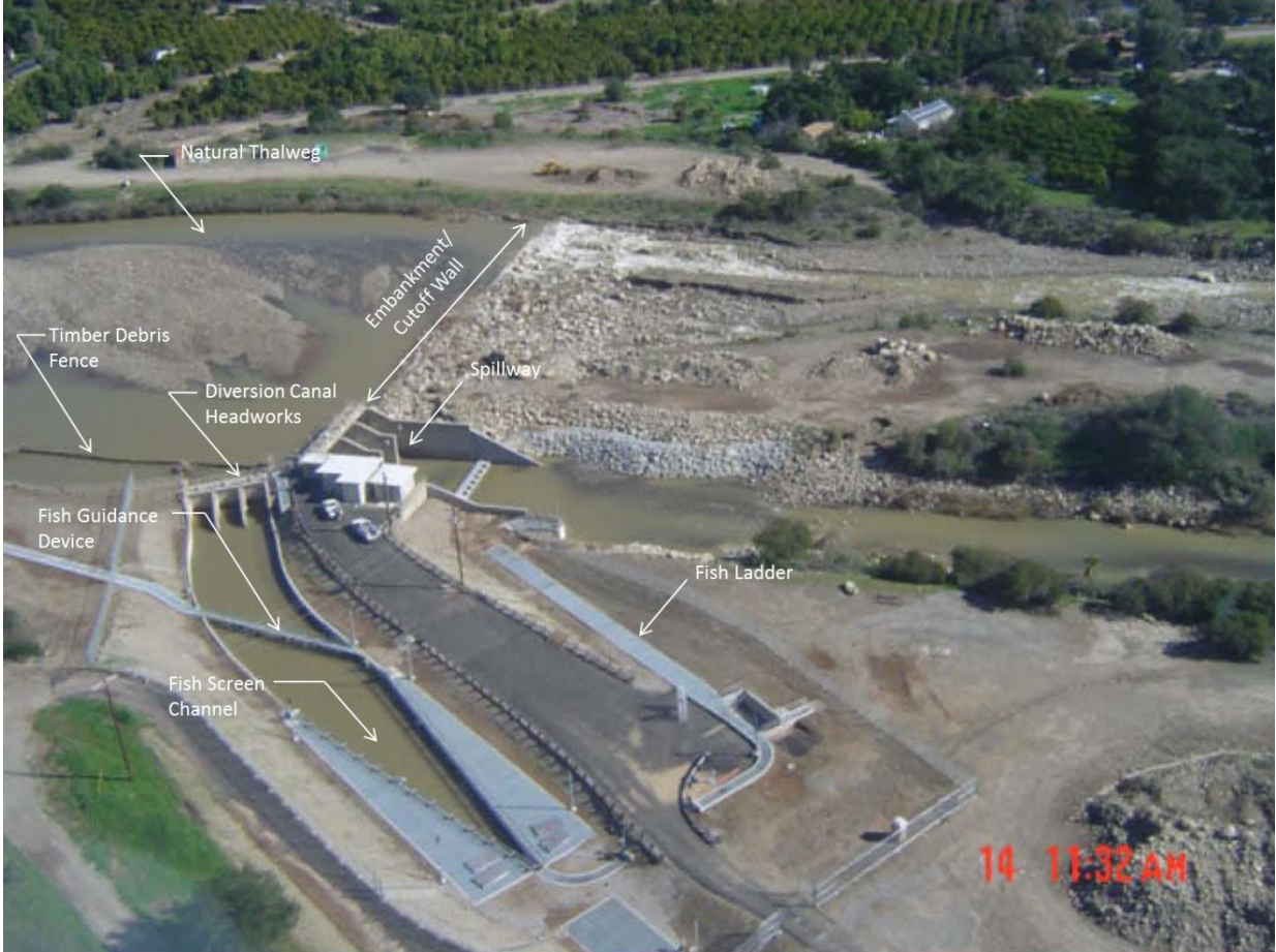
Figure 3. Aerial Photo Showing Major Project Features
