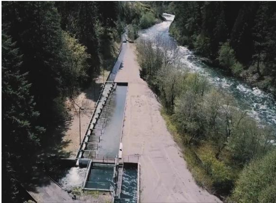
Figure 15. Horizontal Floor Screen (from FCA Website)
