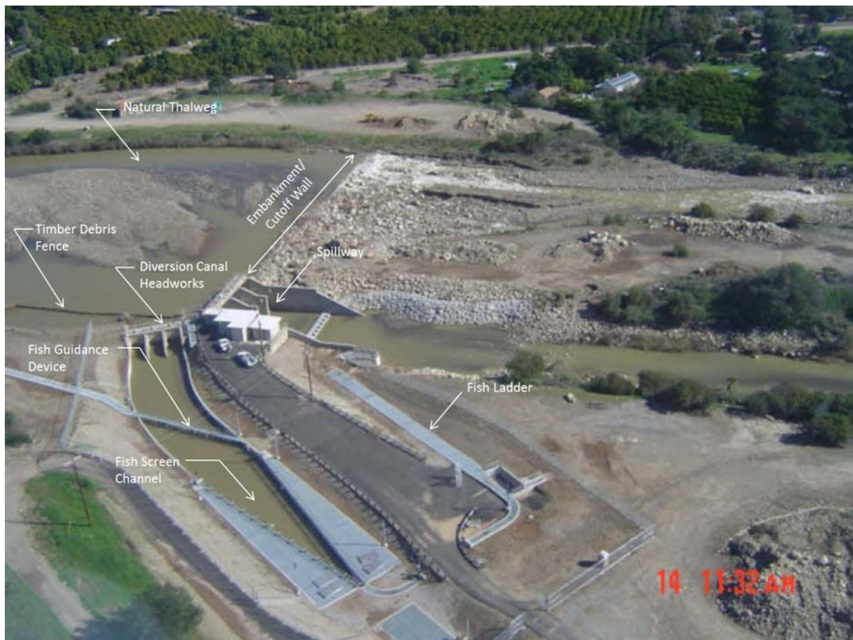
Figure 1-1: Aerial Photo Showing Major Project Features
