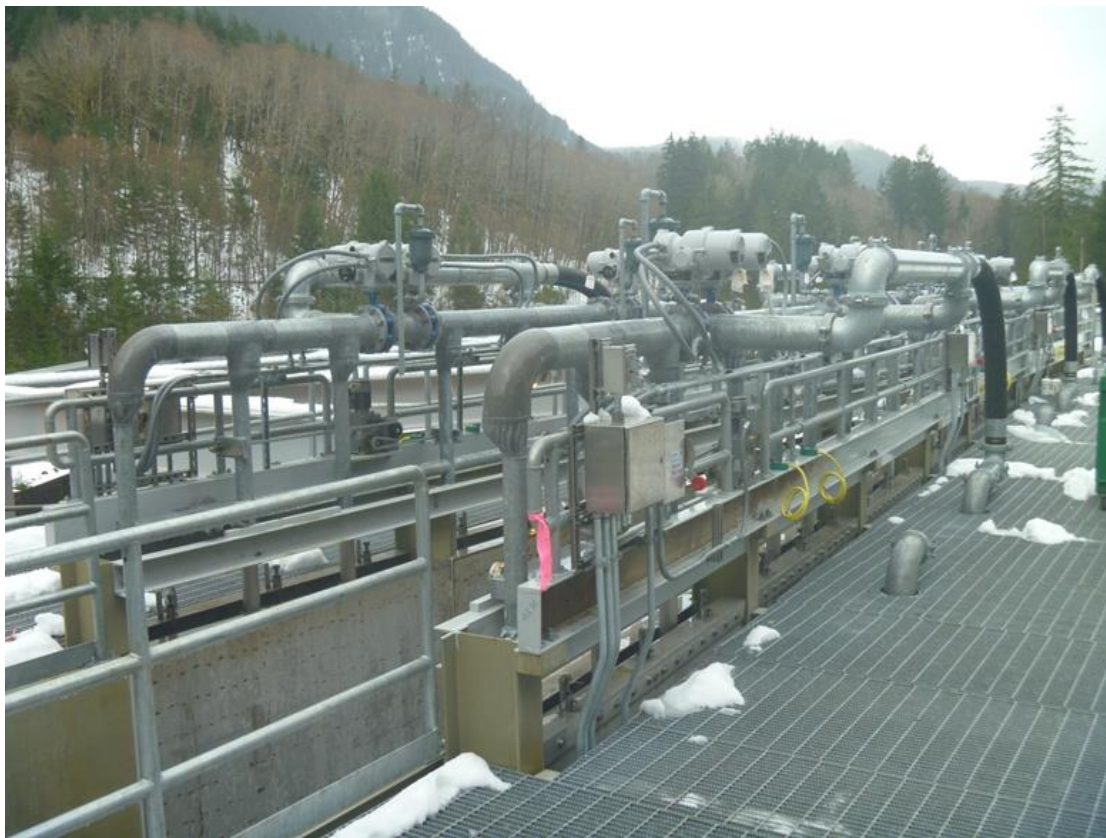
Figure 3-6: Flat Panel Screens with a Water Backspray at the Cowlitz Falls North Shore Collector on the Cowlitz River, Washington (Courtesy Tacoma Power)
