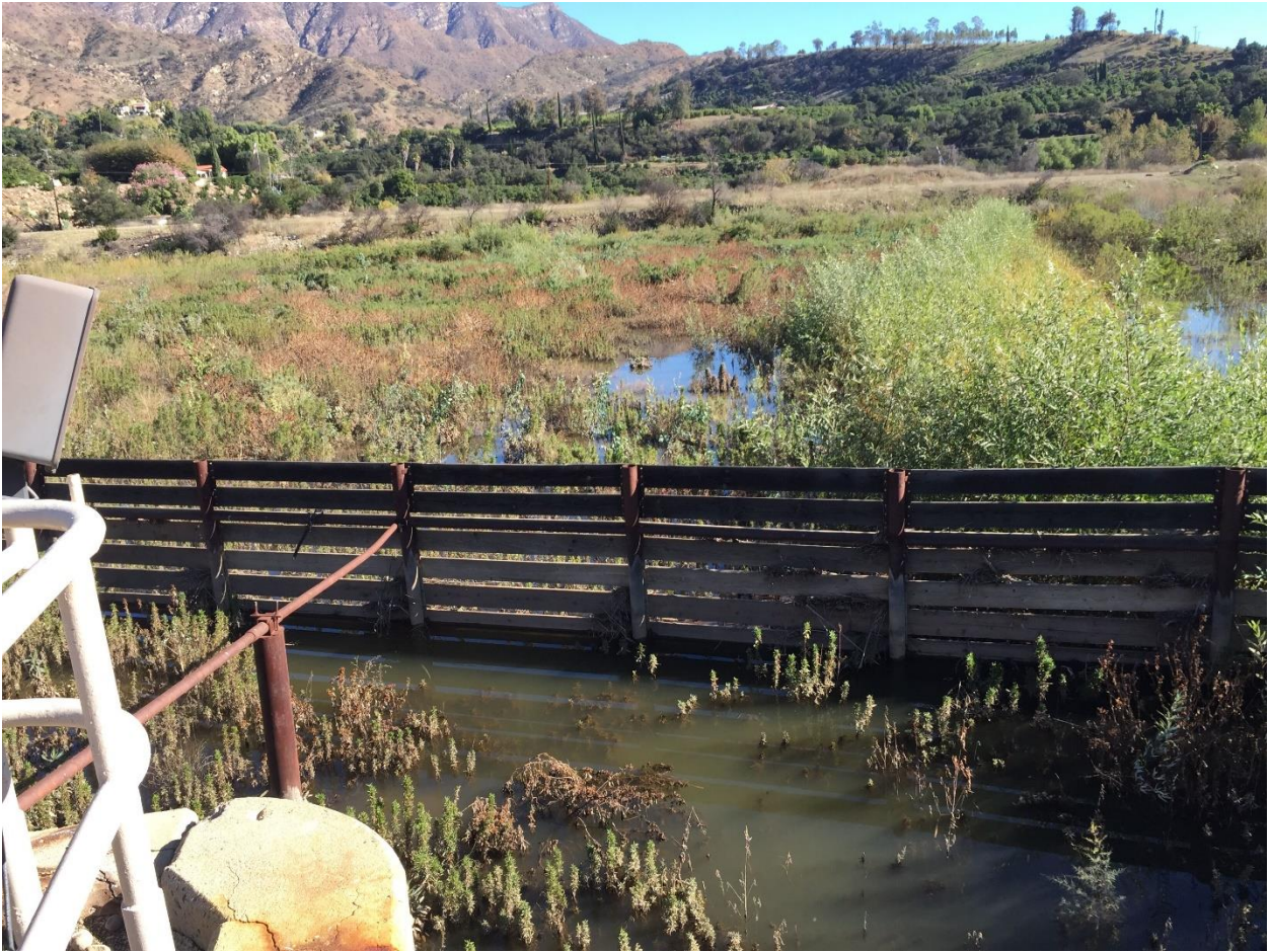
Photograph 6. View looking northeast, of the forebay area and timber debris fence upstream of the Diversion Canal Headworks. Standing water is present from the December 2018 storm events.
