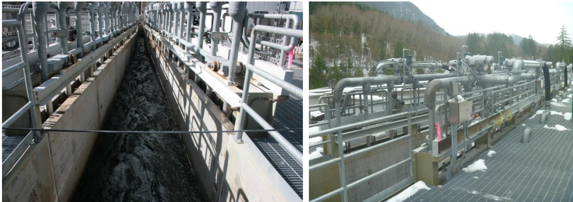
Figure 12. Backwash Carriage and Backwash System Piping (Cowlitz Fall Dam Fish Collection Facility)
